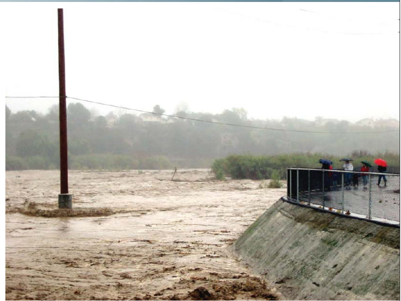
Exposed soil-cement embankment protection withstands flood waters.
